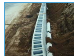
Retaining Wall Drain
